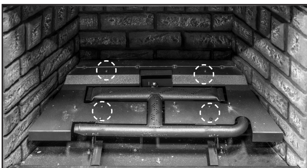
Figure 42: The log grate is removed next by simply lifting it off the grate tabs.
